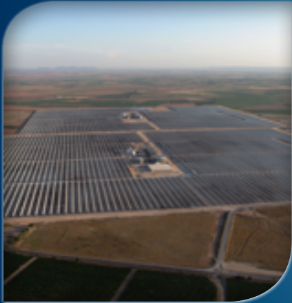
MANCHASOL CONCENTRATED SOLAR POWER PLANT
